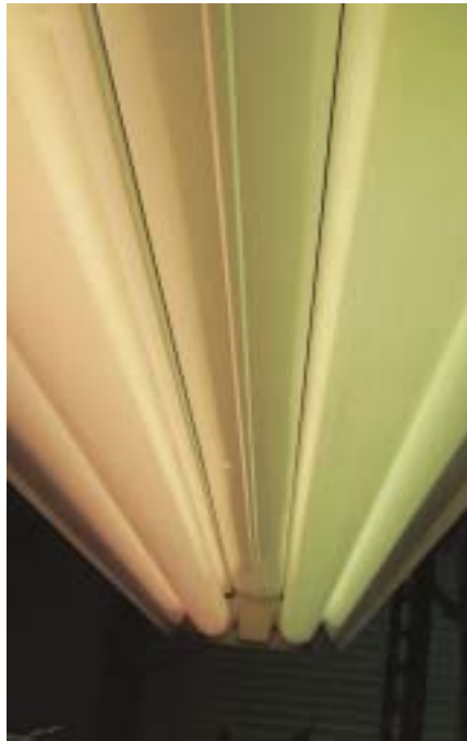
ABOVE Shoplight fixture with alternating warm and cool white 4-foot (1.2-m) long 40-watt bulbs. The bulbs are dated with the installation date and are replaced in rotation (not all at once) after 12 months of operation.
