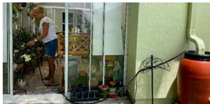
The submersible pump in the rain barrel allows easy watering in the greenhouse
