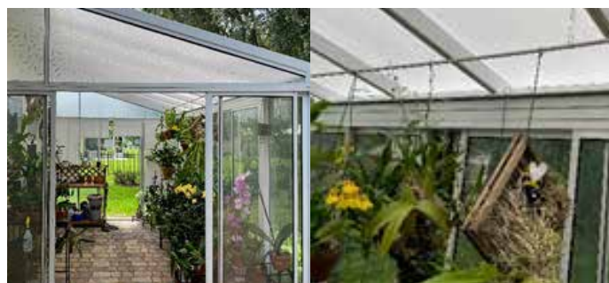
Window film was attached to the upper glass surface to shade plants from too bright sunlight
