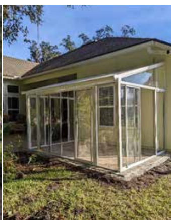
The finished structure attached to the house with sliding doors on the other three sides
