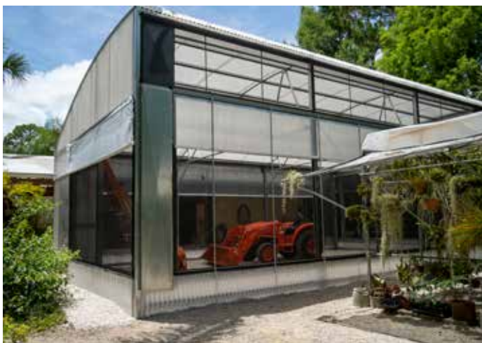
Time for a new greenhouse!
